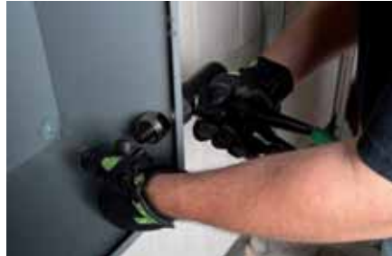
Fix the die and start punching.
