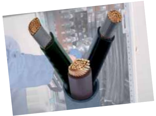
Round-crimping sector sleeves in three steps.
